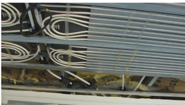
**Figure 6 – Raccordement hydraulique**
