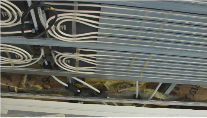
Figure 5 – Raccordement hydraulique
