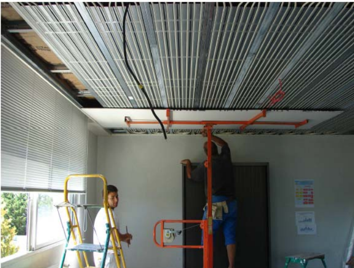
Figure 7 – Pose du parement
