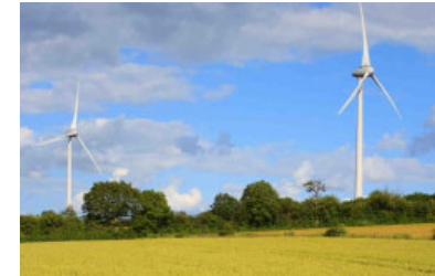
Eolienne Enercon E-82 Saint-Cyr-en-Pail, Mayenne
