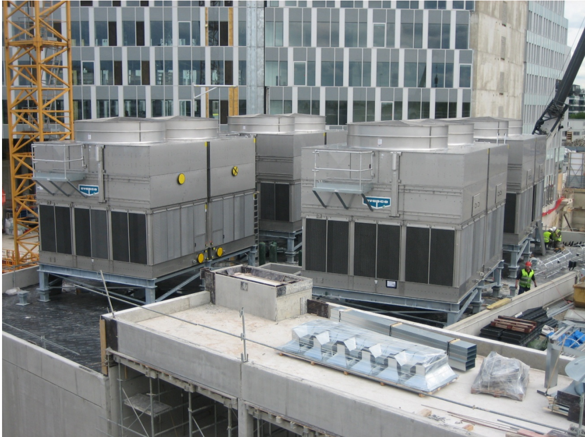
View of the (4) UAT 224-318 double cell cooling towers after rigging
