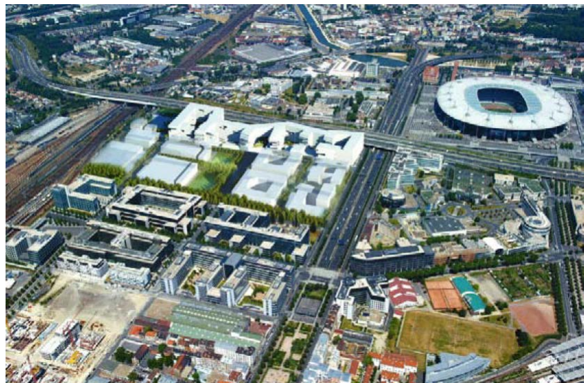
View of the Stadium with the newly built Business district that is cooled by Sesas 3
