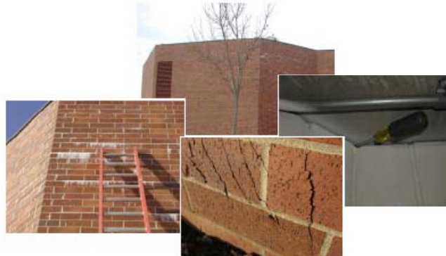
Damage to brick facade of pool building due to lack of specification for (a) sealing of air leakage paths in exterior envelope and (b) balancing to assure negative pressurization of pool area. Large newer middle school.
