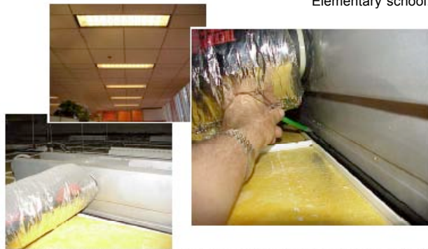
Inadequate cooling and excessive fan power consumption due to poor fit between light troffer diffusers and duct boot provided by a different supplier, allowing up to 25% of flow at diffuser to bypass directly into ceiling plenum. Highrise office tower.
